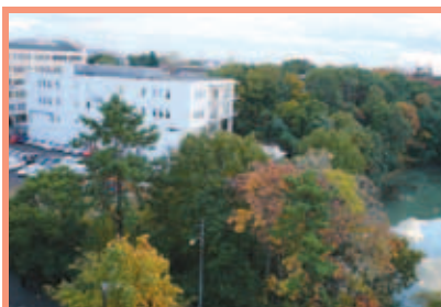
New Student Union Building
